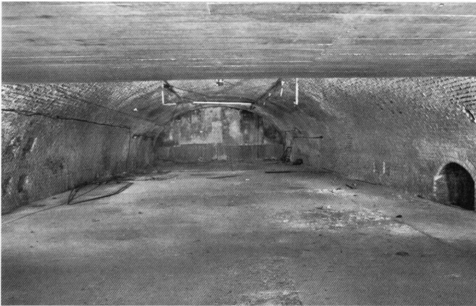
Blackheath Hill Tunnel in March 2008. Photo by Nick Catford
